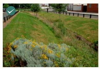
Linear Swale - Key feature of the character area, provides a SUDs solution to drainage and wetland habitat running through the heart of the development.
